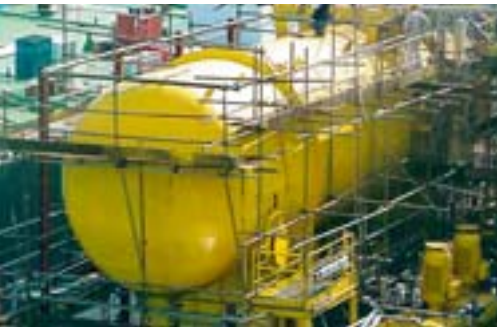
Even at remote locations: the LEWA service is available at any time and all over the world
